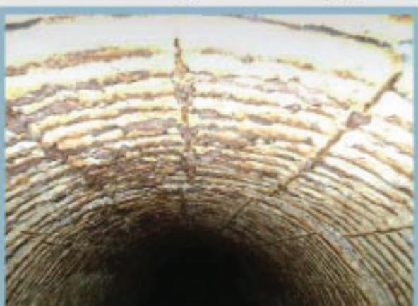
H<sub>2</sub>SO<sub>4</sub> Gazı Etkisi İle Beton İçindeki Donatı Çıkmış
